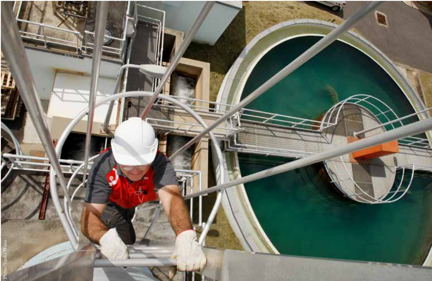
Drinking water plant in Montauban, France.
